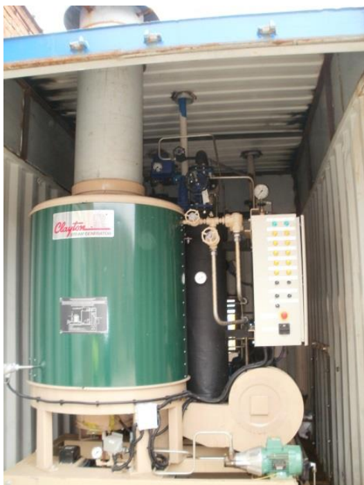
Fig. 1 - Clayton Steam Generator IB-3 E0-80-1M SKID in the container
